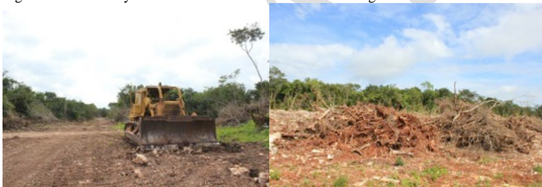
Figure 15. Machinery used for deforestation for commercial agriculture.
